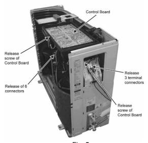
Fig. 5 7. Remove the 4 screws of the Electronic Controller.
